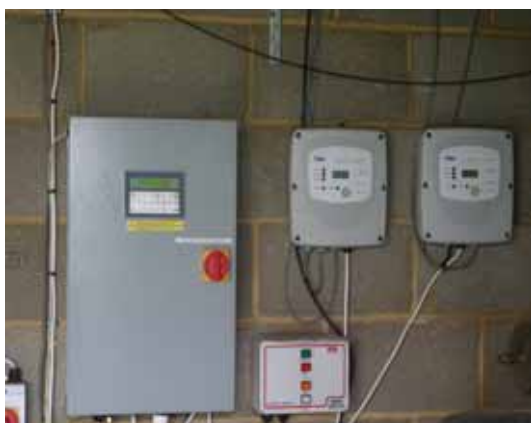
FIG. 1. CONTROL EQUIPMENT FOR BIOFRESH ETHYLENE CONTROL SYSTEM.
