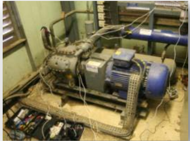
Figure 3.6.6 - Compressor wired for ClimaCheck monitoring
