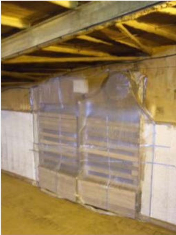
Figure 3.5.3 - Main door sealed inside
