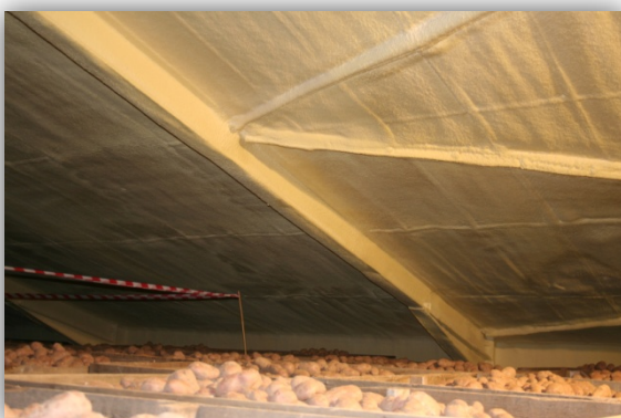
Figure 3.7.1 - Spray foam insulation
