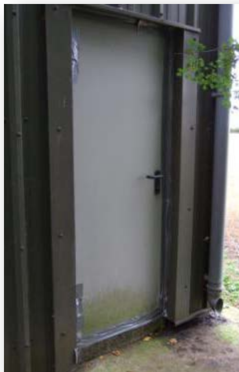
Figure 3.5.8 - Personnel door sealed outside
