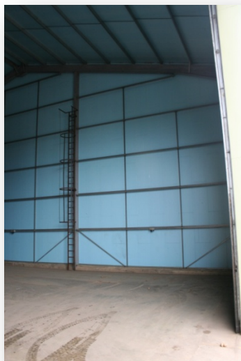
Figure 3.7.2 - Styrofoam board insulation
