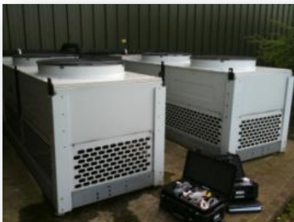
Figure 6.5.5 - Remote condenser/compressors
