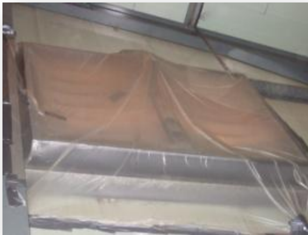
Figure 3.5.3 - Main door sealed inside
