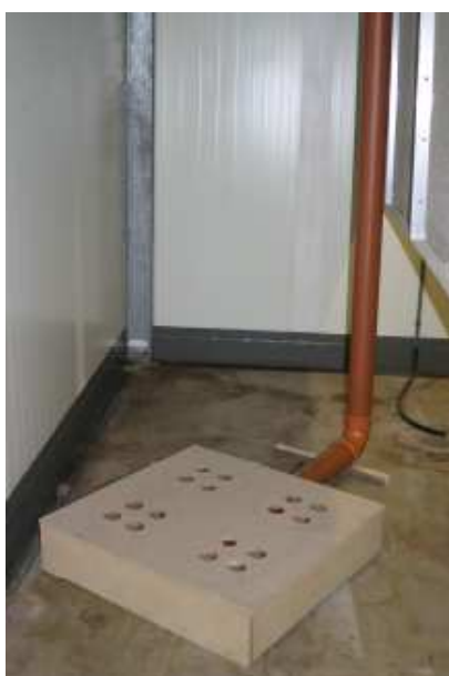
FIGURE 1. MANIFOLD, SUPPLIED WITH CLEAN AIR FROM A CIPC UNTREATED STORE, FOR SUPPLYING AIR TO 4 'PILES' OF POTATOES.
