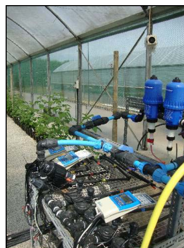
Figure 3. The Galcon timers used to control irrigation. Photo taken on 9 July 2010
