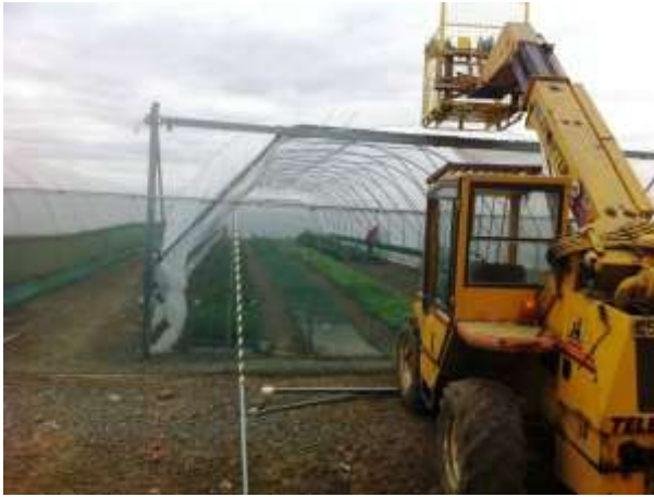
Figure 1. Bay 1 of the Centre's 'ProTech' tunnel.
