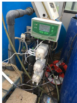
Figure 26 IntelliDose controller installed at the deep pool facility using three peristaltic pumps, one each for the A and B tank and acid supply.
