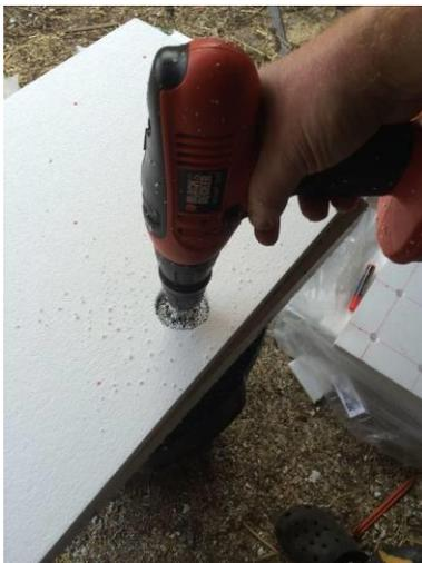
**Figure 3.** Drilling out the 50 mm air gaps.
