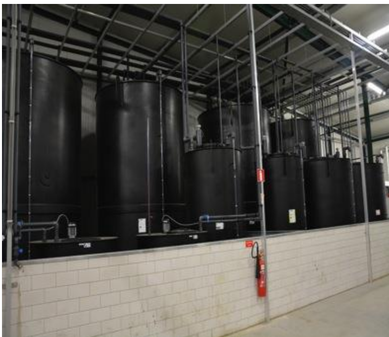
Figure 9. Nutrient stock tanks for a 10 hectare tomato nursery (Holland, 2014)
