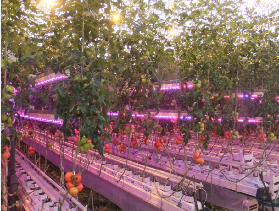
Figure 3: An example of inter-lighting with LED for lighting a tomato crop. Here two sets of LED fittings are being used in conjunction with overhead HPS lighting
