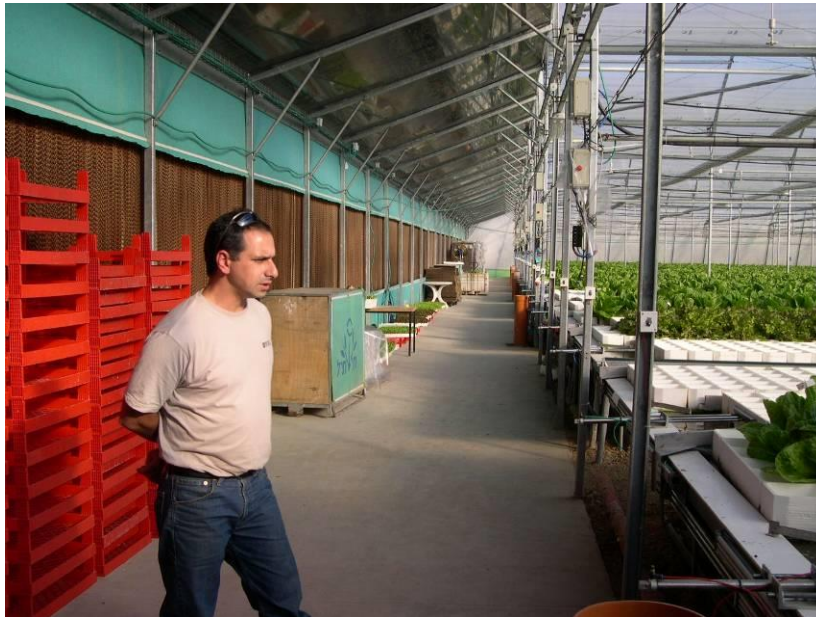
Plate 5: General view along the house, noting the evaporative cooling and shading above to assist workers during harvesting and other in-crop operations.
