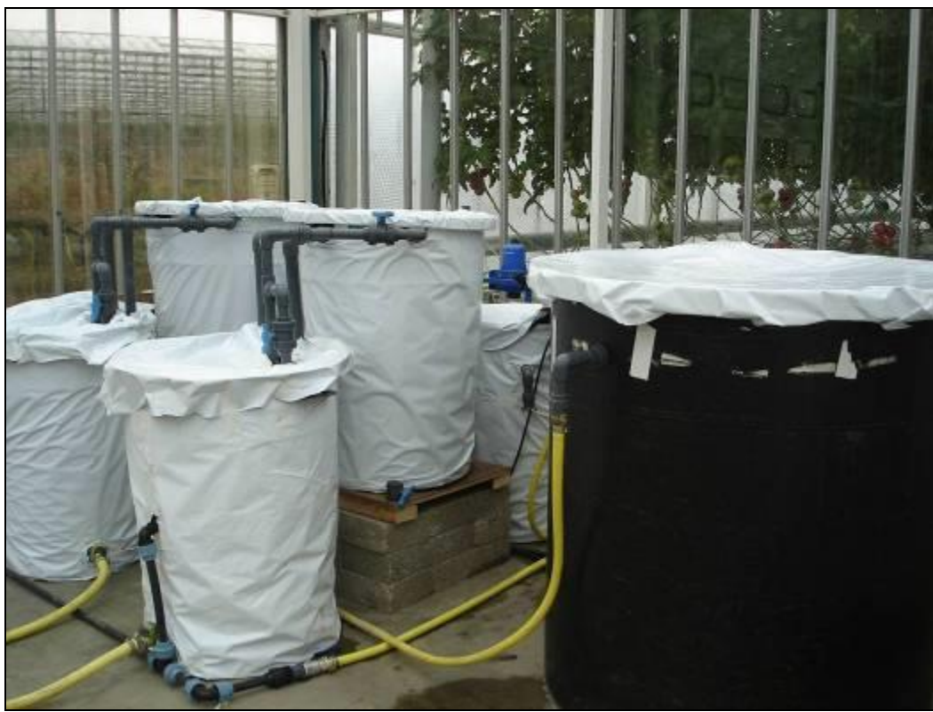
Plate 4. Slow sand filter at Nursery B
