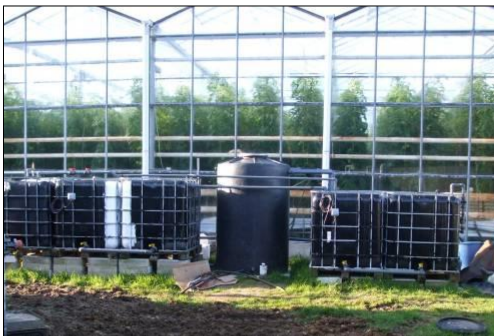
Plate 3. Slow sand filter arrangement at Nursery A
