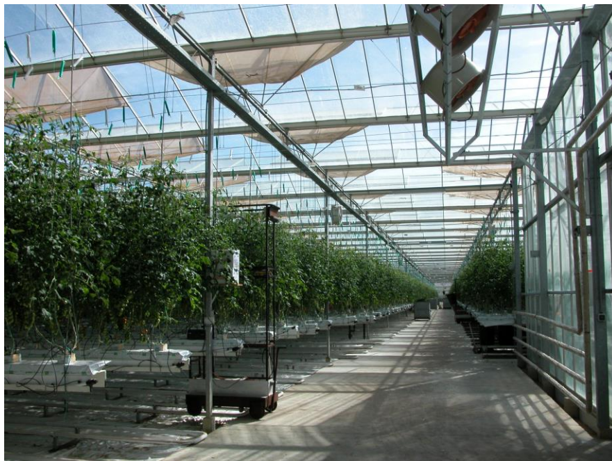
Figure 5. Example of outward facing fans directed towards the double door entrance of a Spanish glasshouse. These fans switch on automatically when the door begins to open and continue to run until it is closed.
