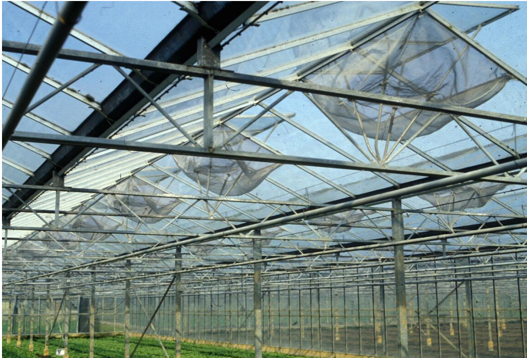
Figure 2. Screened ventilators on the commercial nursery
