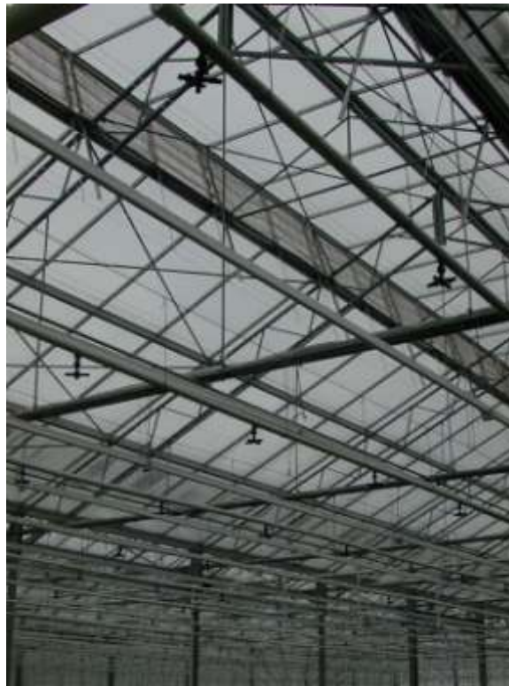
Plate 4.2. Misting systems to cool air temperature in Holland.
