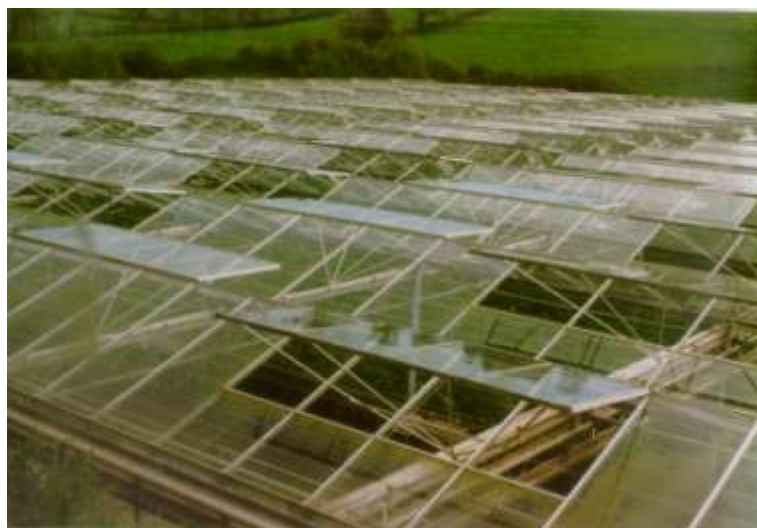
Plate 4.1. Ventilation on glasshouses in southern England.
