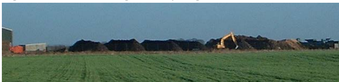
Figure 1 – The Site at Organic Recycling Ltd
