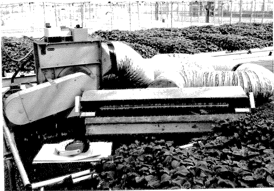
Plate 2. Detail of the air delivery orifice
