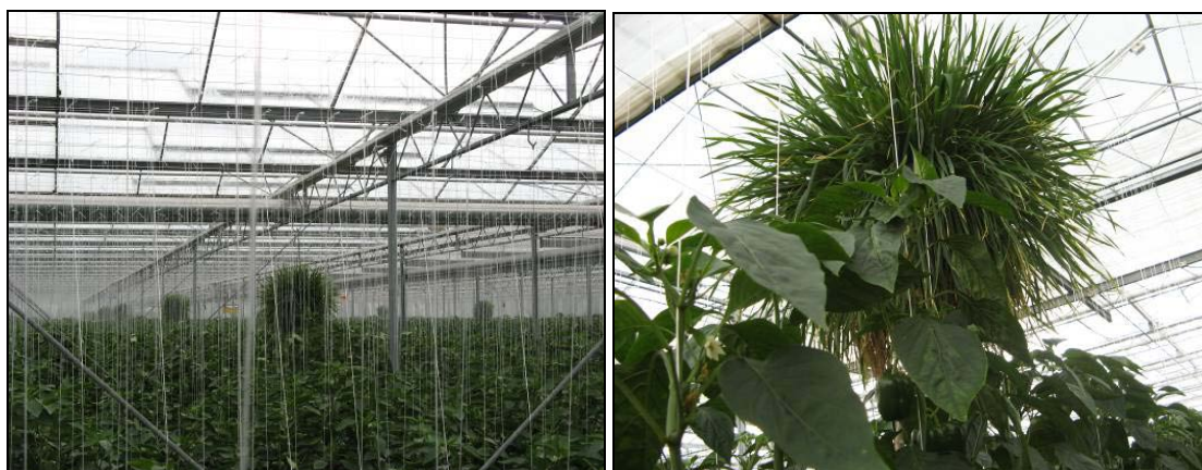
Figure 25. ORUs in place above the pepper crop (left) and close up of a single unit (right) in week 8, 2010.
