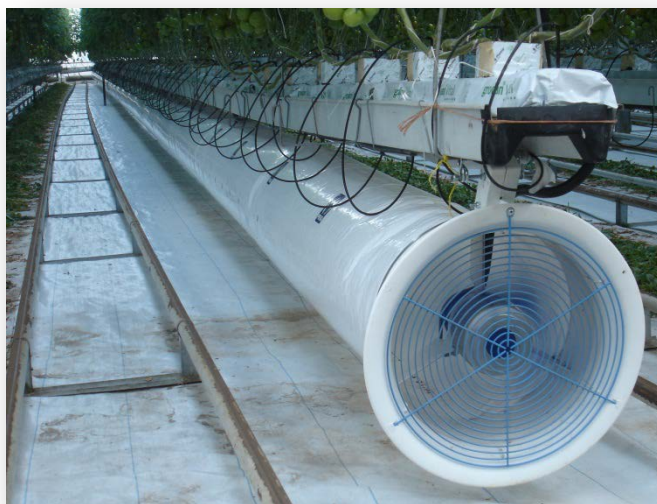
Figure 18 – Simple fans and ducts installation
