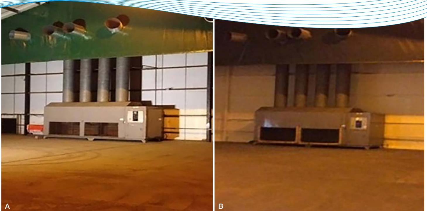
Figure 1. Store with newly installed air dividers (A) and newly applied spray foam insulation (B)
