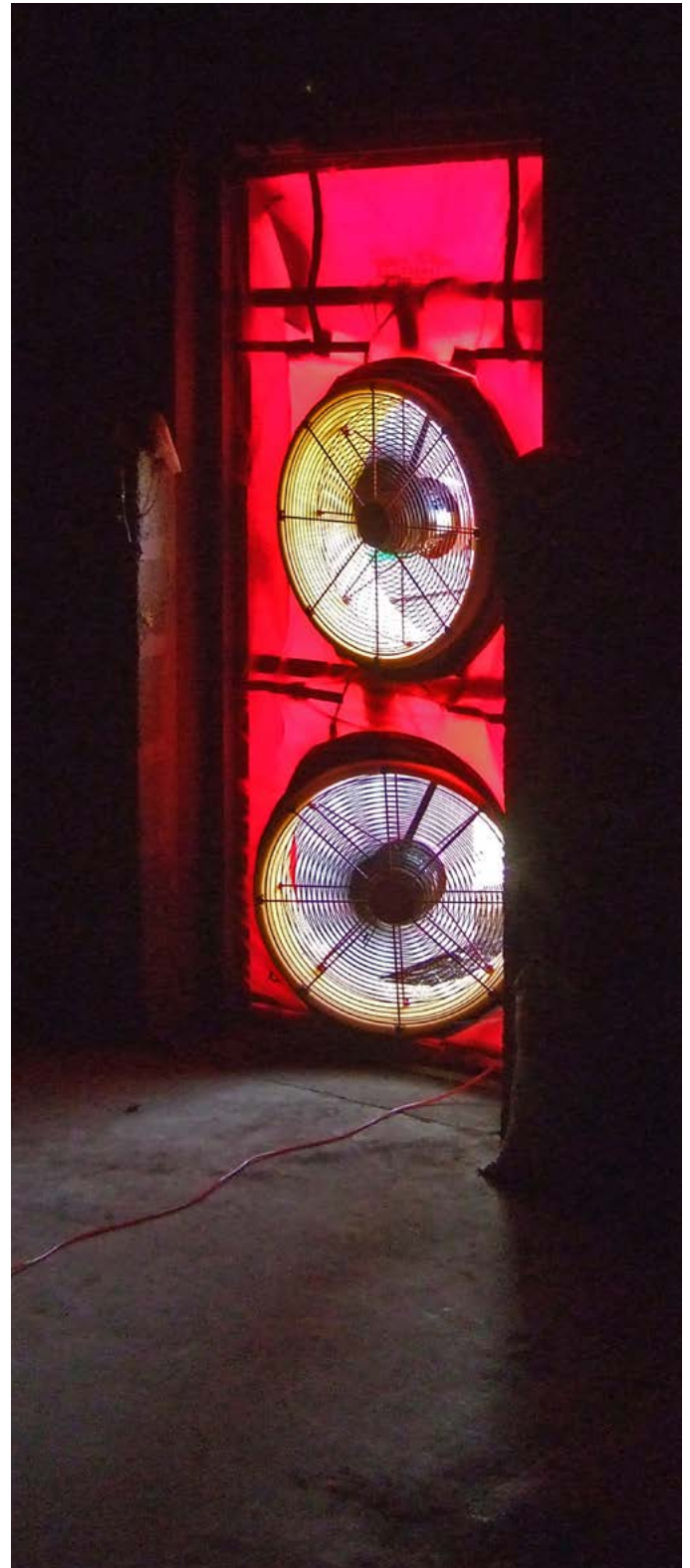
Figure 1. Air leakage assessed by forced introduction of air and monitoring pressure change
