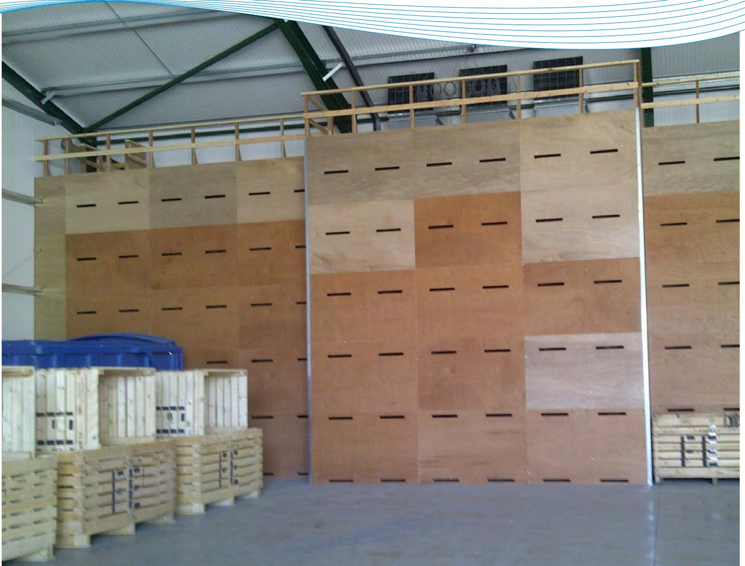
Figure 1. Example of a suction wall with 'letterbox' openings, providing a non-positive drying system
