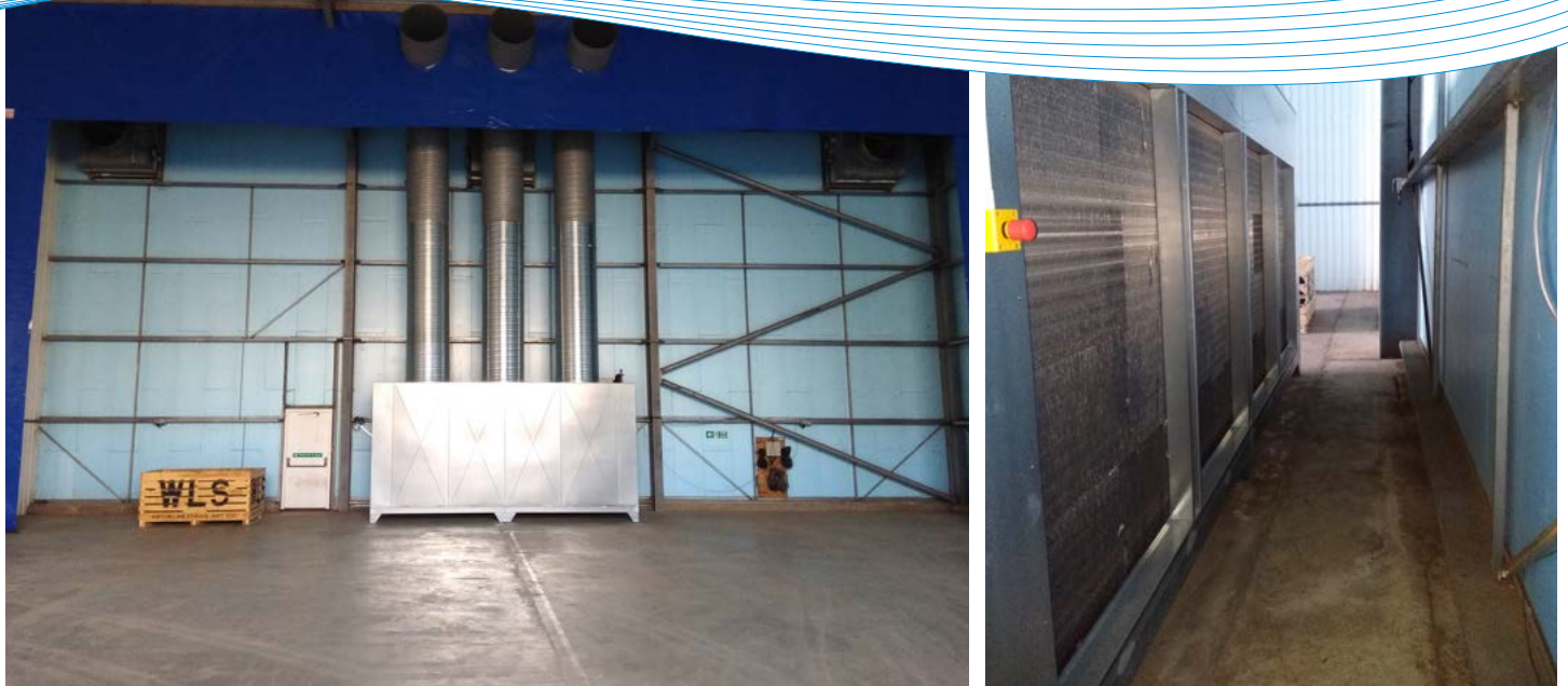
Figure 1. Commercial testing 180° turned fridge unit in overhead throw store at WLS. The unit was turned so the evaporators face the store wall rather than the boxes
