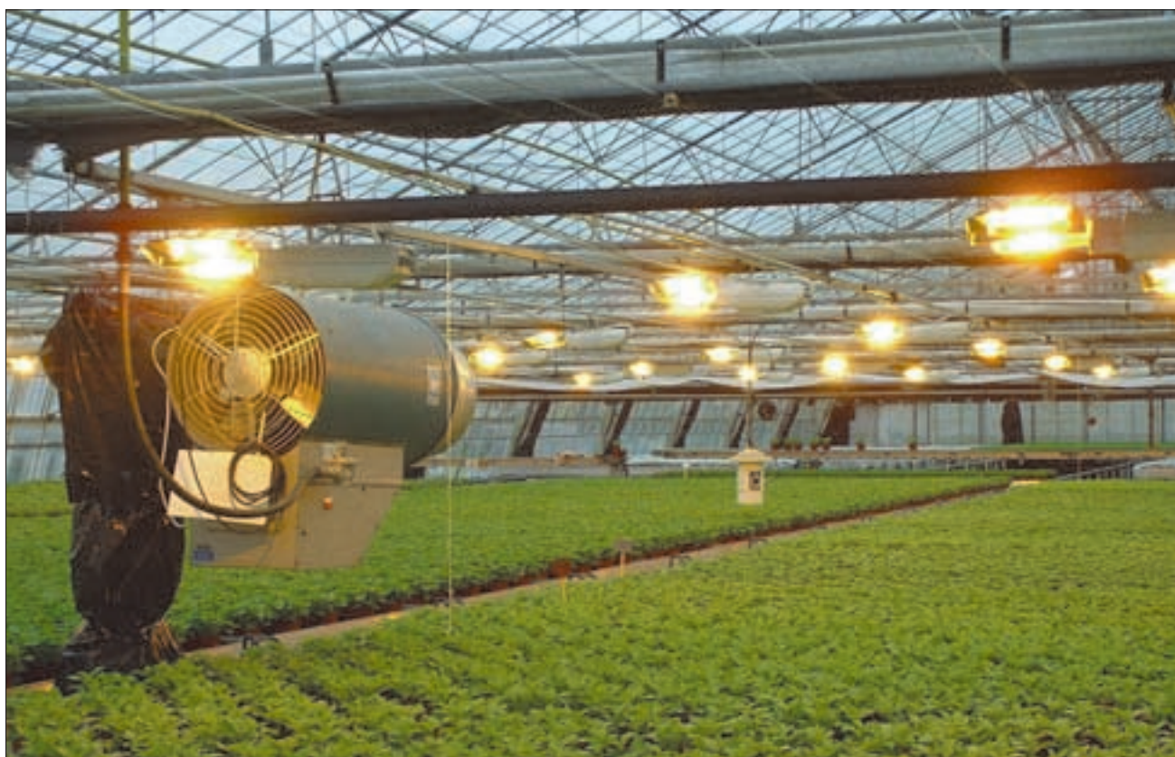
Use fans to keep air moving over the plant surface
