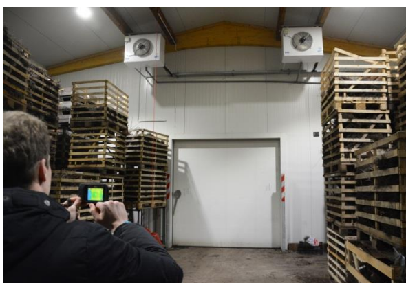
View of the cold store door, with two evaporators above it with a normal and an infra-red heat imaging camera.
