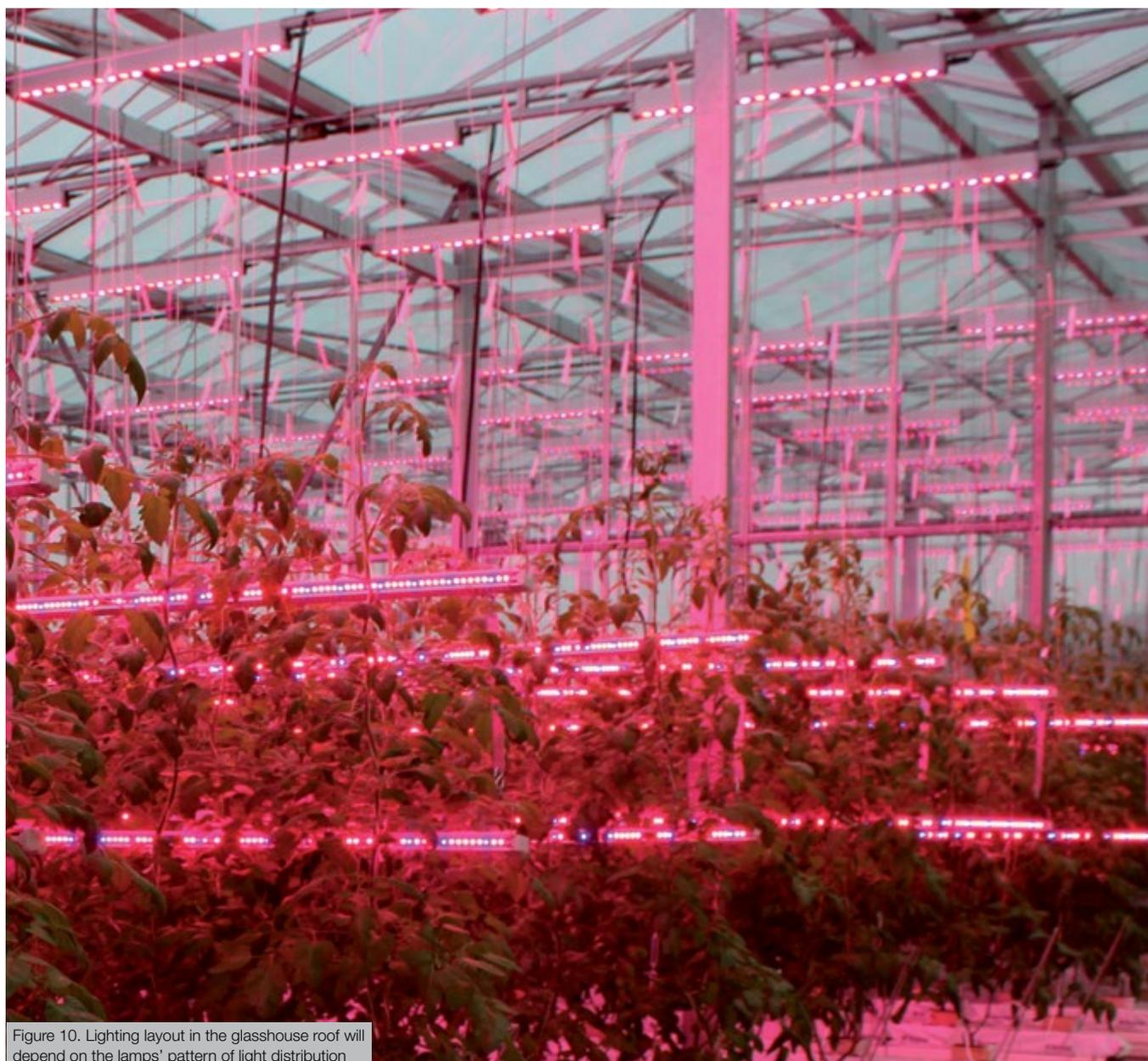
Figure 10. Lighting layout in the glasshouse roof will depend on the lamps' pattern of light distribution
