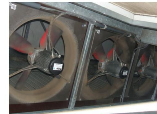
Fig 25 Cooling fans in ambient stores require an output equivalent to 30 room volumes per hour
