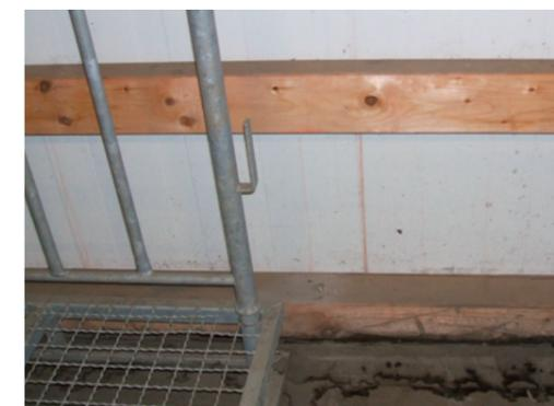
Fig 43 Safety barriers on internal walls help to prevent damage from machinery and crates
