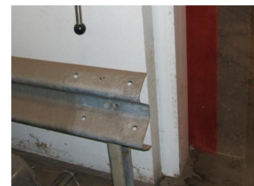
Fig 44 Safety barriers on external walls help prevent damage from forklift trucks and other machinery
