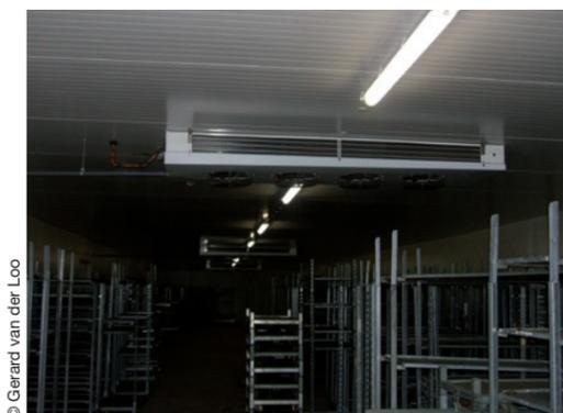
Fig 12 A direct cooled store is used to hold cutting material and to store rooted cuttings in plug trays prior to despatch
