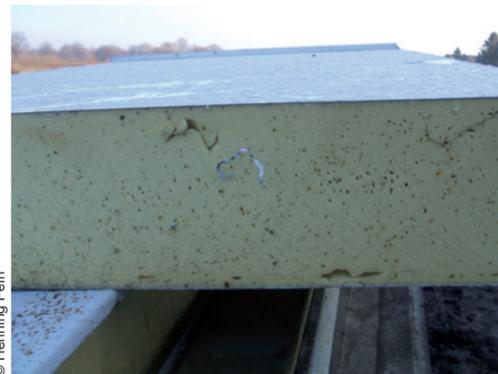
Fig 31 Typical insulation foam used in cold store
