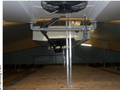
Fig 30 Cooling chamber above storage space of jacketed store. A thin aluminium sheet separates the cooling system from the store, so preventing desiccation. Low temperatures pass through the aluminium sheet into the store beneath.
