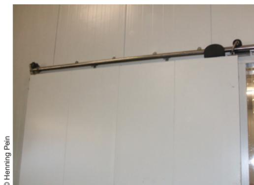
Fig 32 Some sliding doors have a positive sealing action
