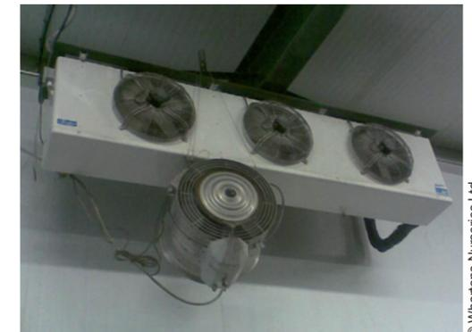
Fig 15 Mist atomisers provide direct cooling and unlike fogging units, enable clear vision when working
