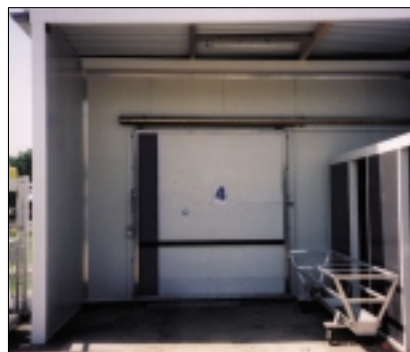
7 A chilling unit set at an interim temperature could be used to prevent 'chilling injury'
