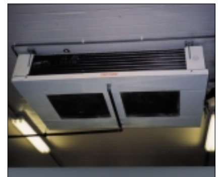
8 Avoid placing cut flowers directly beneath cold store refrigeration units in order to reduce potential water loss
