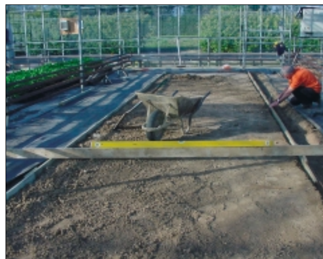
6 Construction of prototype capillary flow beds which have potential for use in the UK
