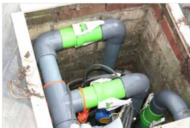
35. Tray plant field drainage sump with submersible pump
