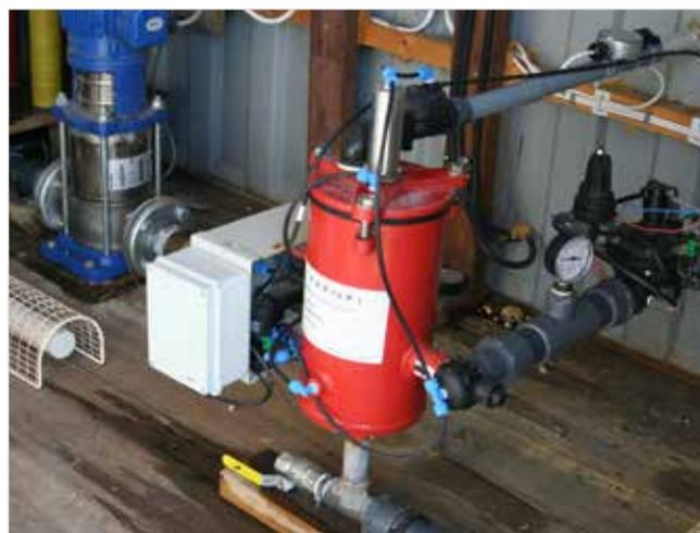
49. Small disc filter for final water filtration
