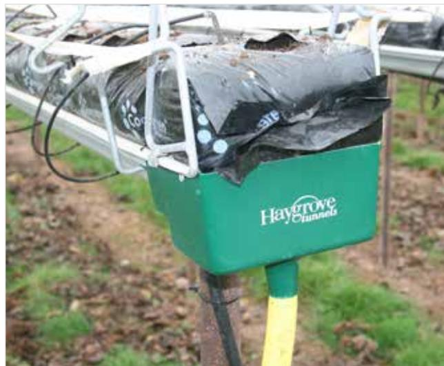
8. End cap and downpipe for gutter systems in multi-bay tunnels
