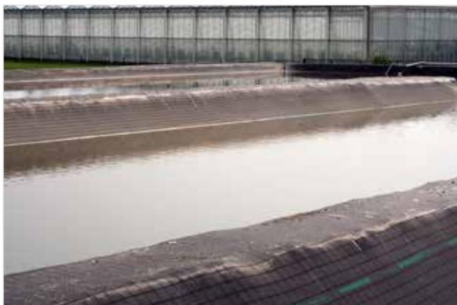
1. Roof water collection reservoir on a strawberry farm in the Netherlands, with separate sections for roof water and drainage water
